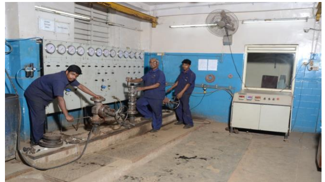
Hydro Testing Setup
